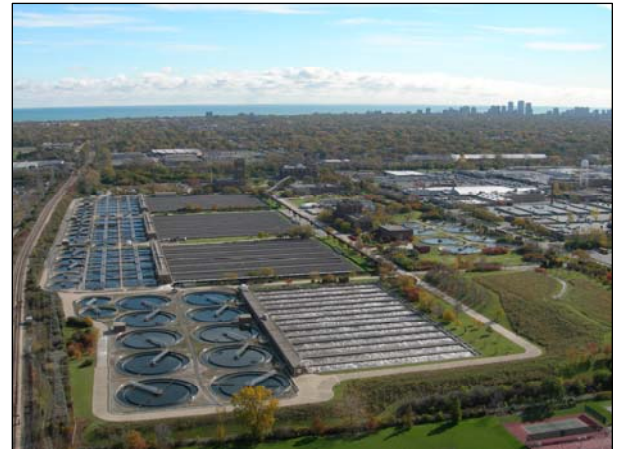
Wastewater treatment plant. Photo: Greater Chicago Reclamation District.
