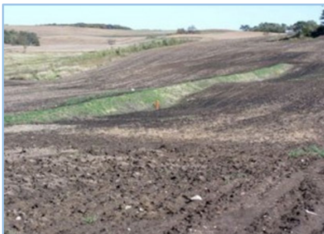
Lenawee Conservation District in Michigan installed a combination of practices including grassed waterways (left) and water and sediment control basins (right).
