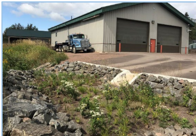
Cook County SWCD installed rain garden and bioswale projects which improve local stormwater management and capture sediment.
