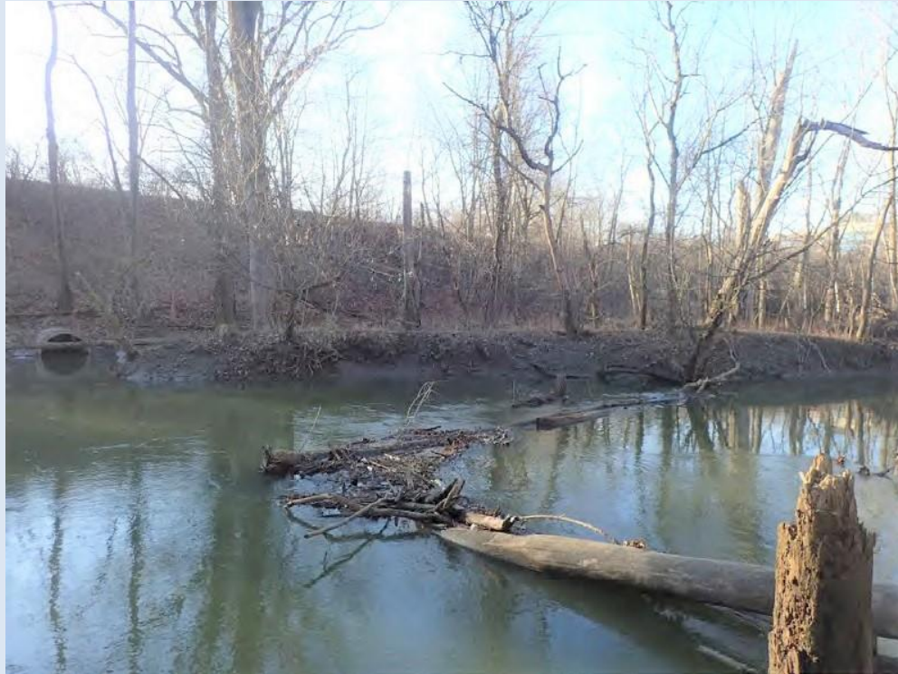
Eroding streambank on Swan Creek
